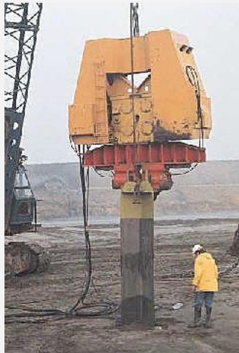
Akin to dynamic compaction, vibro-compaction densifies and stabilizes in-situ soil conditions. In vibro-compaction applications, this is achieved by a vibrating head attached atop a large vertical steel ram.
